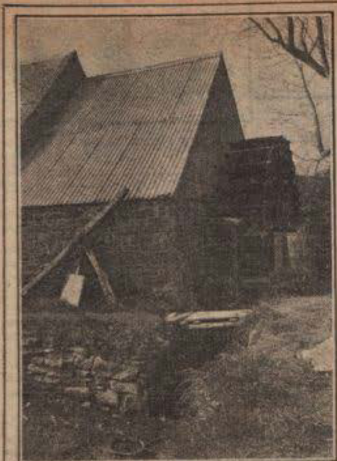
THE OLD WATER-WHEEL of the woolen yarn factory at Llanrhystyd, in Cardiganshire.
